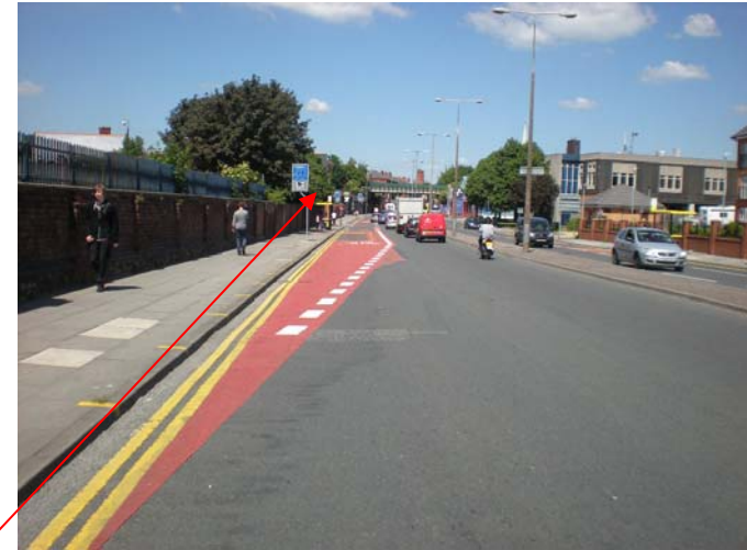
Rice Lane, just north of junction with Hornby Rd, commencement of bus lane entry taper 2
